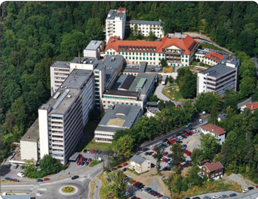
The Norwegian Radium Hospital in Oslo.
