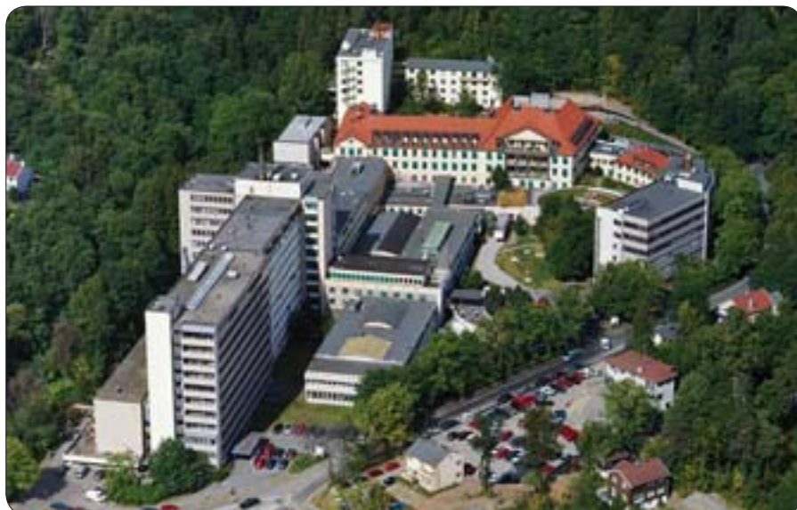
The Norwegian Radium Hospital in Oslo.
